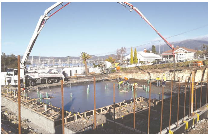
Progress on the Anchorage Development
